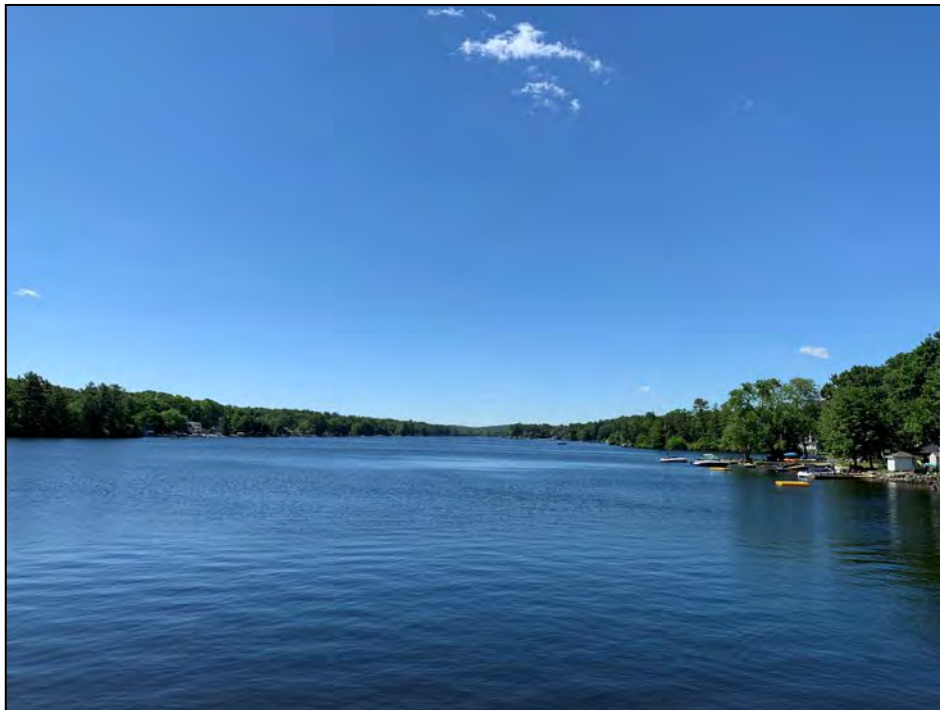
Photo No. 2: Impoundment overview from the dam crest.
