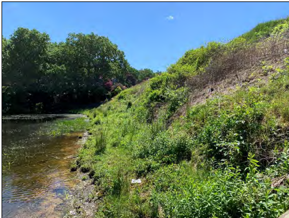
Photo No. 13: Downstream slope from the low-level outlet looking right.
