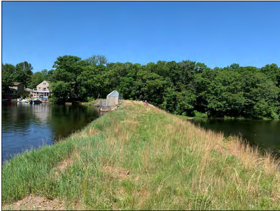
Photo No. 11: Crest from the right abutment looking left.
