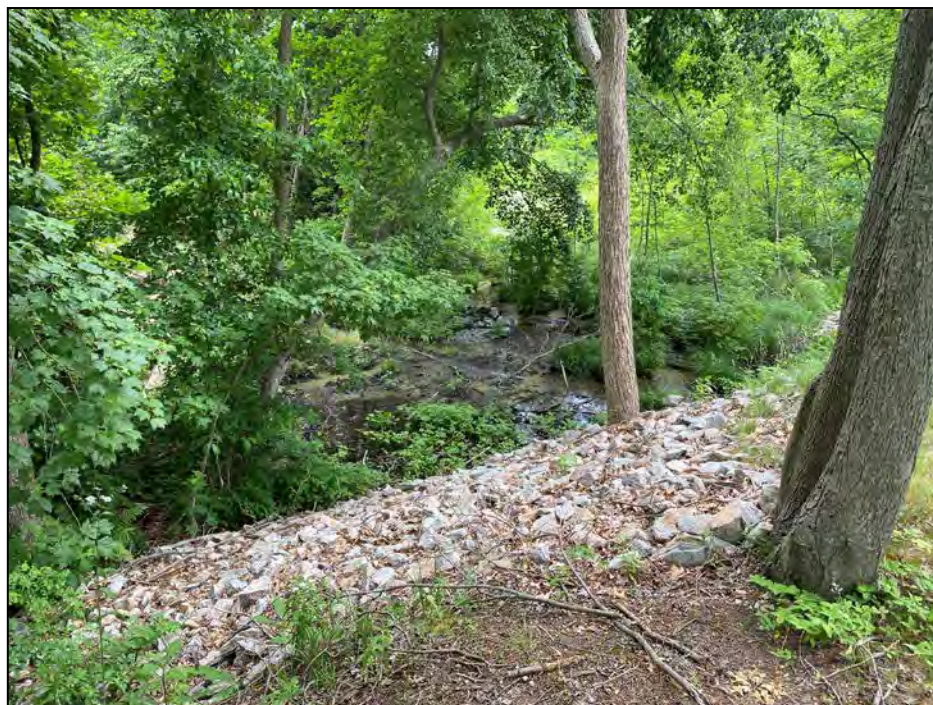
Photo No. 38: View of the area downstream of the dike. Note ponded water and wetland type vegetation.
