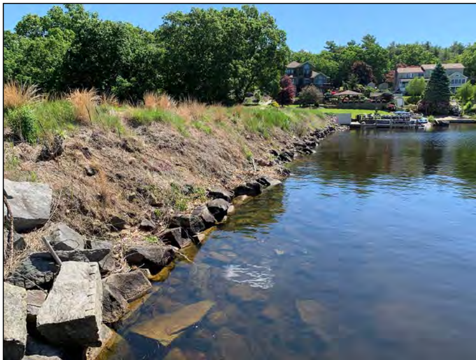
Photo No. 6: Upstream slope right of the low-level outlet. Note bare soil throughout the slope.
