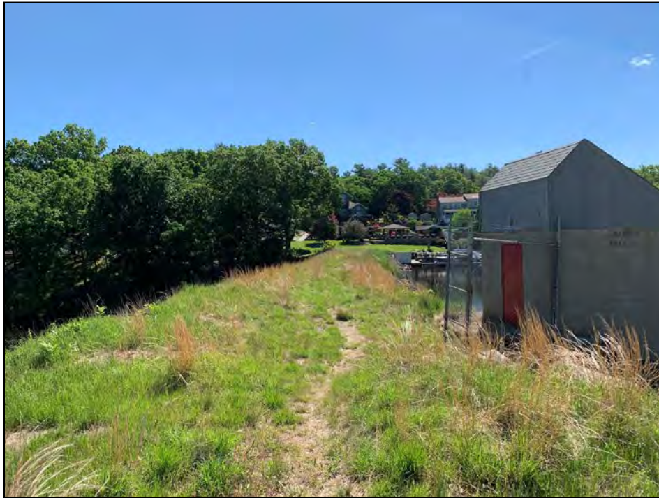
Photo No. 9: Crest from the low-level outlet looking right.
