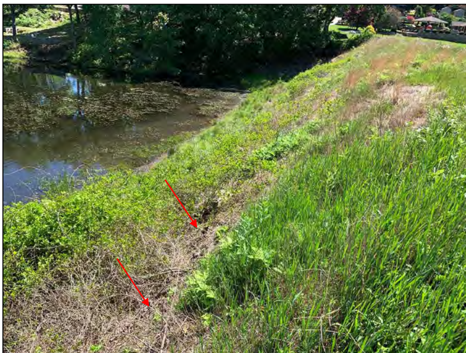
Photo No. 14: Pair of animal burrows (arrows) located 50 feet right of the low-level outlet.
