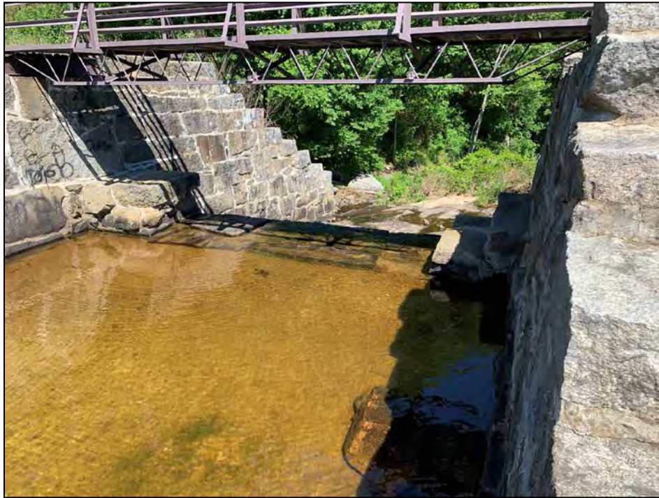
Photo No. 21: Spillway control section.
