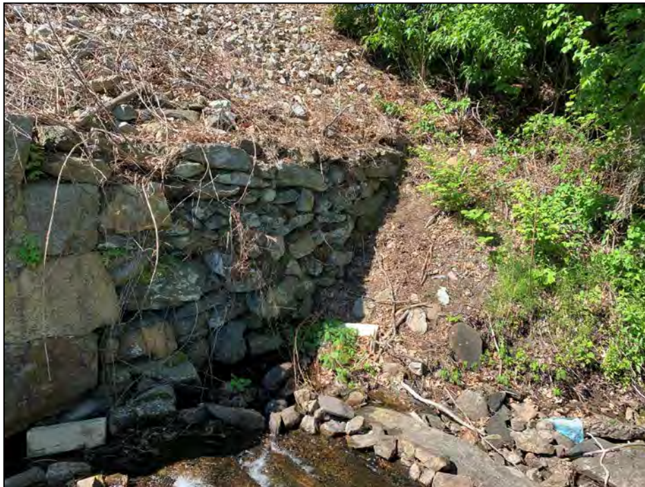
Photo No. 12: Downstream wall and downstream slope left of the spillway.
