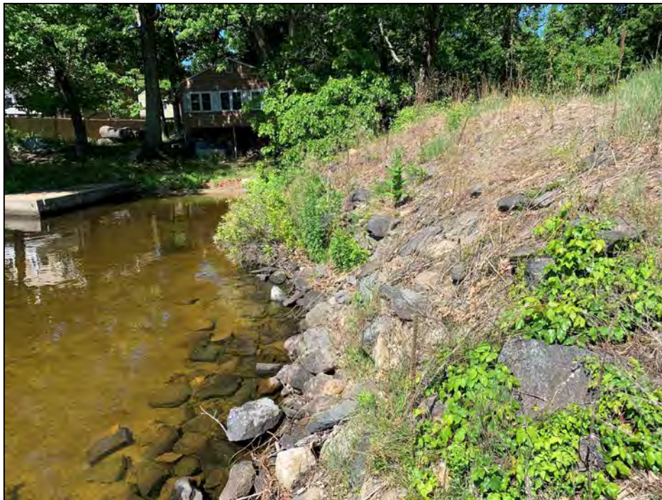
Photo No. 4: Upstream slope left of the spillway.
