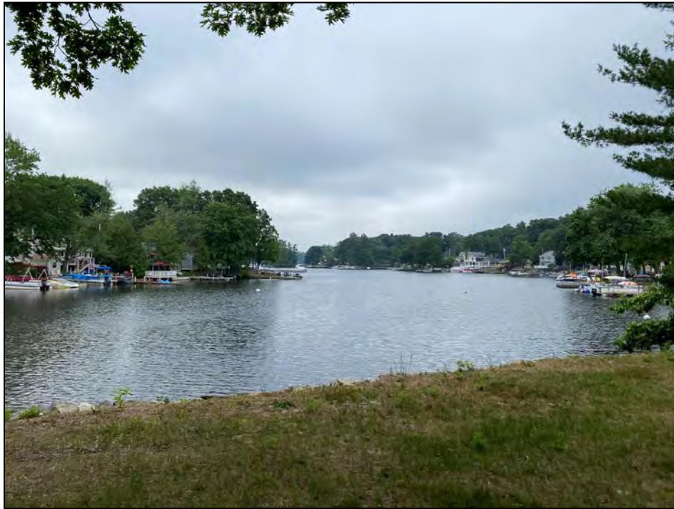
Photo No. 29: Impoundment from the dike crest.
