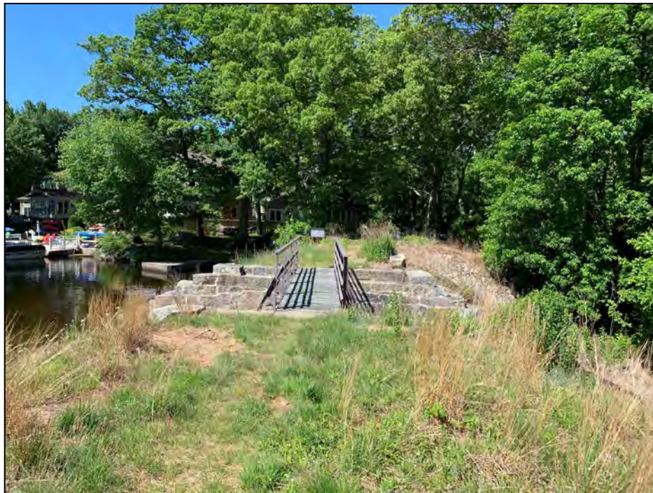
Photo No. 8: Crest from the low-level outlet looking left.
