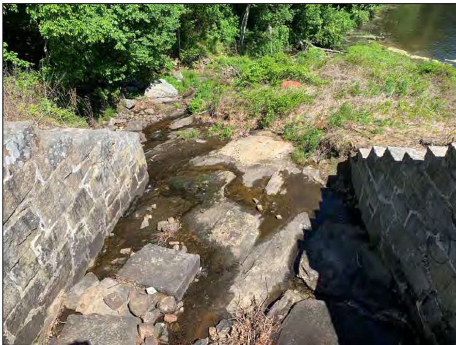
Photo No. 25: Discharge area of the primary spillway.
