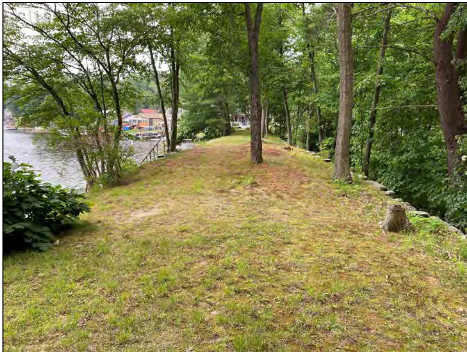
Photo No. 32: Dike crest from right abutment looking left.
