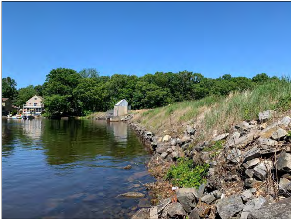
Photo No. 7: Upstream slope from the right abutment.
