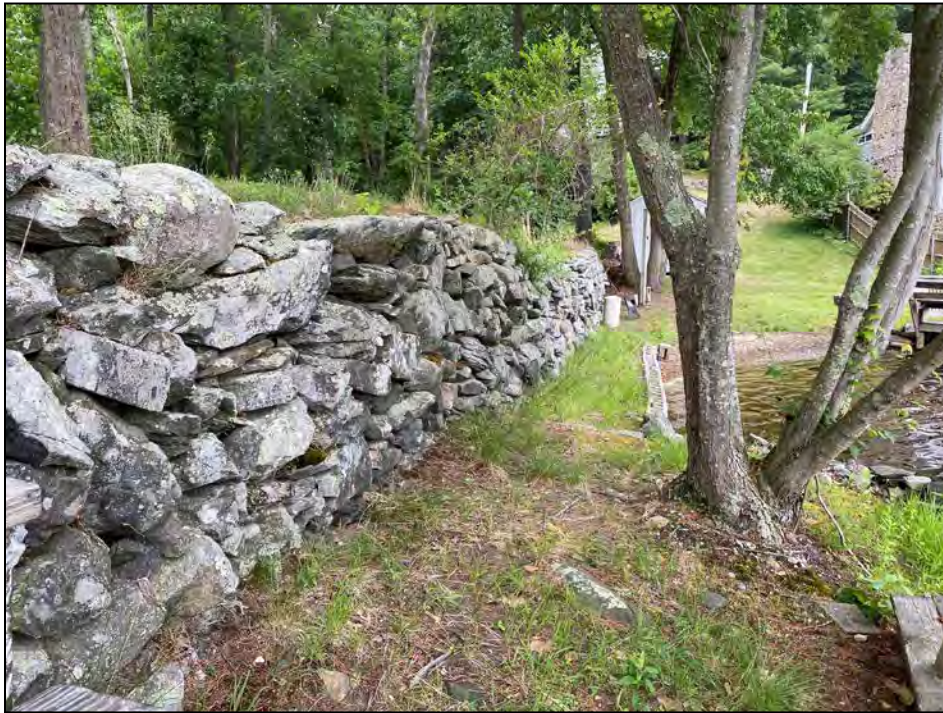
Photo No. 31: Upstream face of the dike from mid-length looking right.
