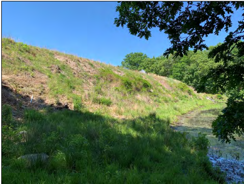
Photo No. 18: Downstream slope from the downstream right abutment looking left.
