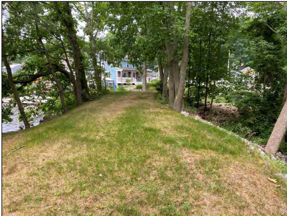
Photo No. 34: Dike crest from near the left end looking left.
