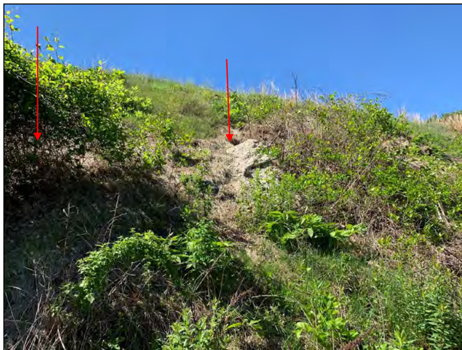
Photo No. 16: Pair of animal burrows (arrows) located approximately 100 feet from the right abutment.
