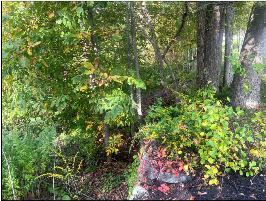
Photo No. 35.: West Dike - Downstream side as viewed from near STA D0+00 looking right.
