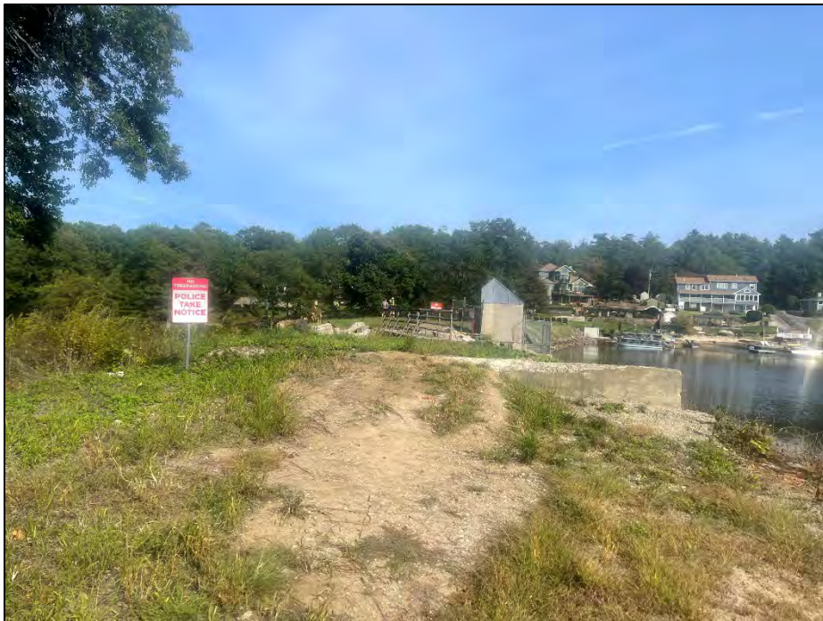
Photo No. 6.: Crest as viewed from the left abutment.
