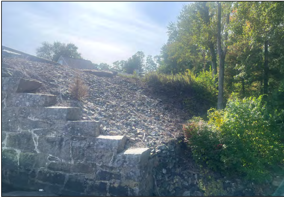
Photo No. 11.: Downstream slope as viewed from the primary spillway discharge channel looking left.
