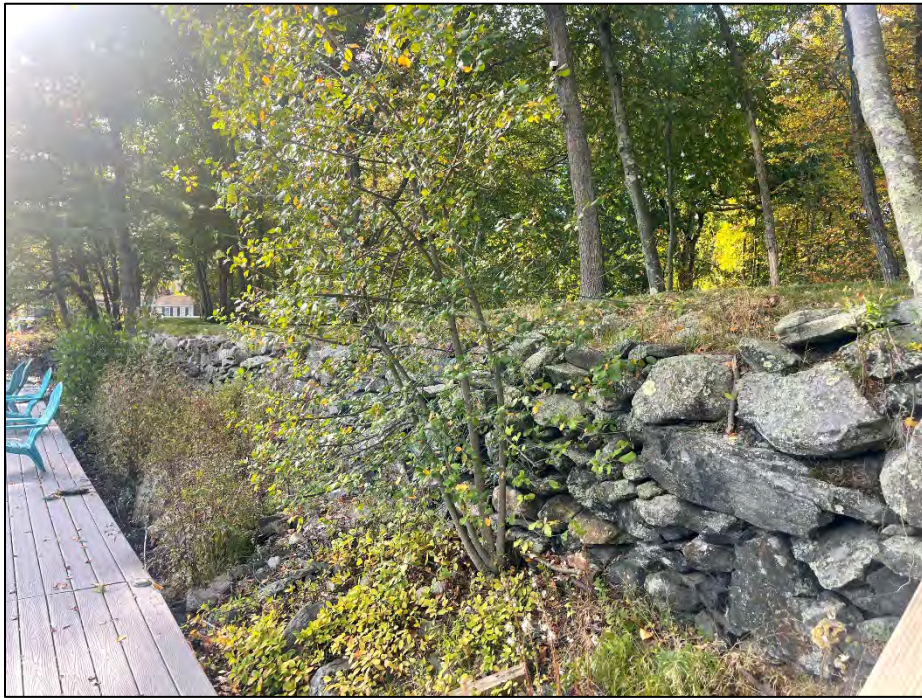
Photo No. 29.: West Dike - Upstream side as viewed from near STA 1+75 looking left.
