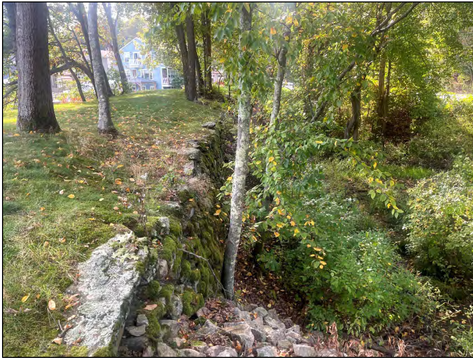
Photo No. 37.: West Dike - Downstream side as viewed from near STA D0+90 looking left.
