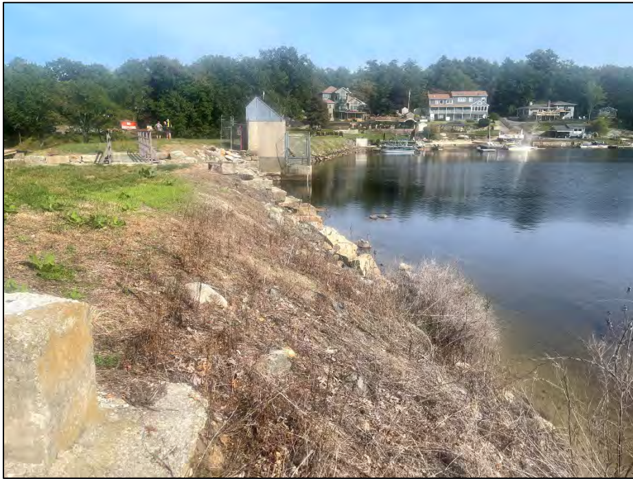
Photo No. 1.: Upstream slope as viewed from the left abutment looking right.
