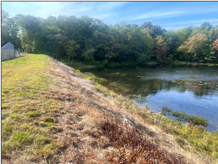
Photo No. 8.: Crest and downstream slope as viewed from near STA 3+00 looking left.
