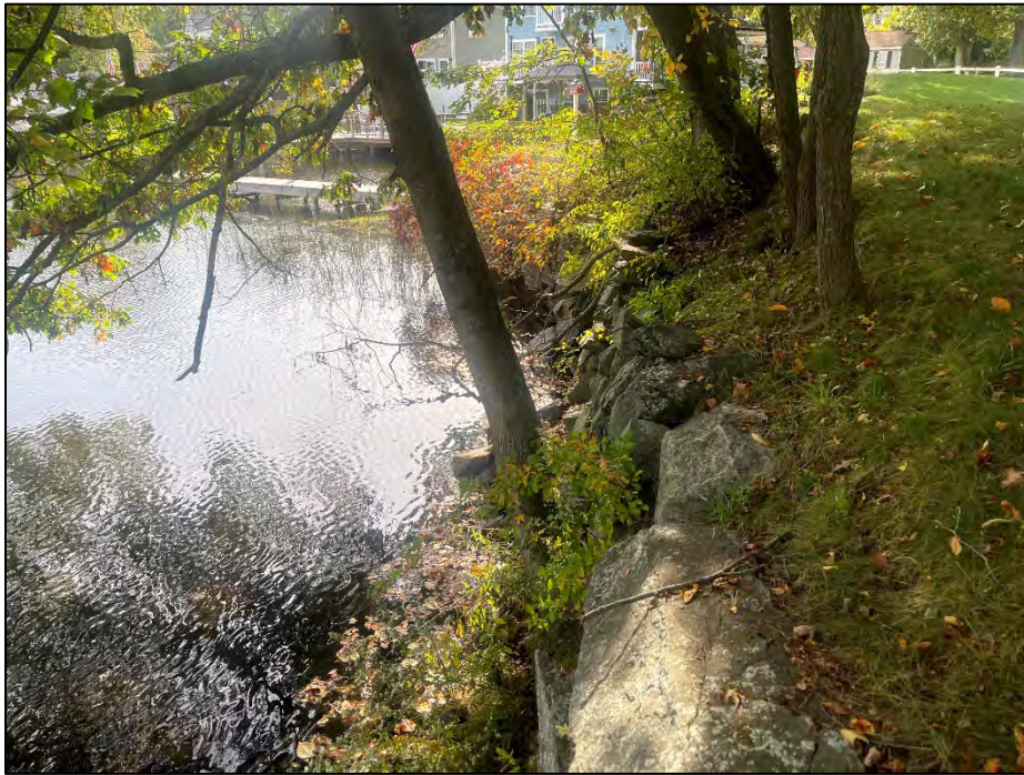
Photo No. 27.: West Dike - Upstream side as viewed from near STA 0+90 looking left.
