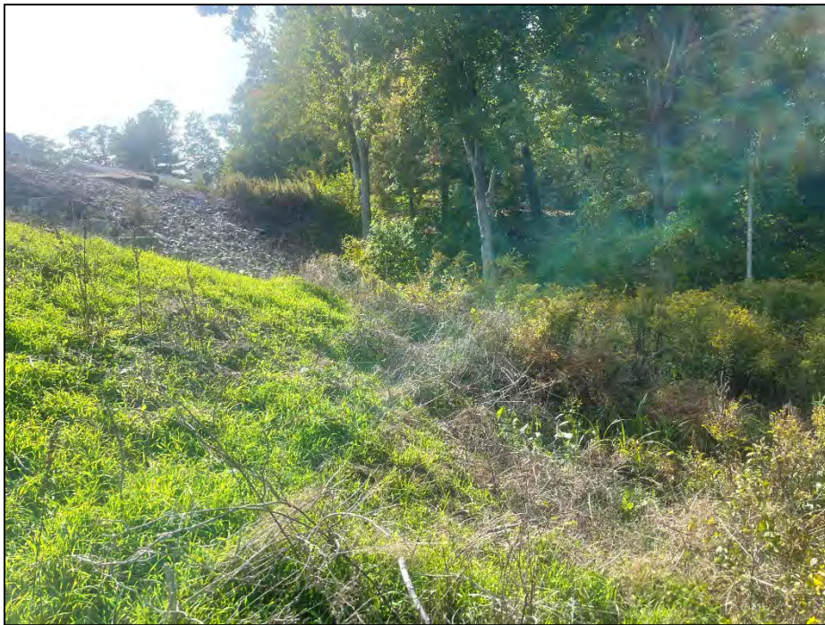
Photo No. 12.: Downstream slope as viewed from near STA 1+00 looking left. No riprap was observed up to the primary spillway; however, no erosion is noted.
