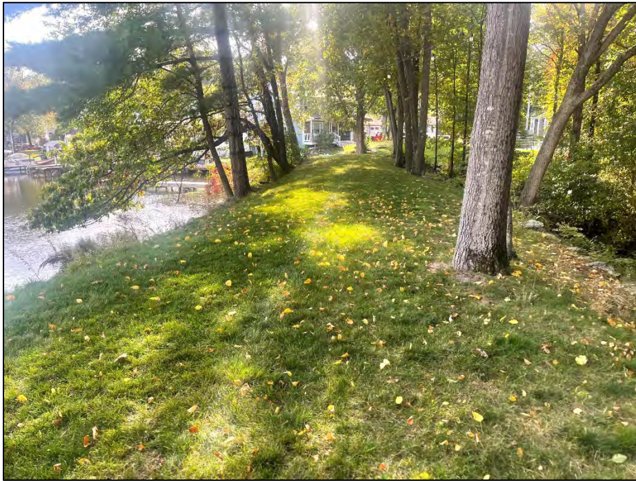
Photo No. 33.: West Dike - Crest as viewed from near STA D1+00 looking left.
