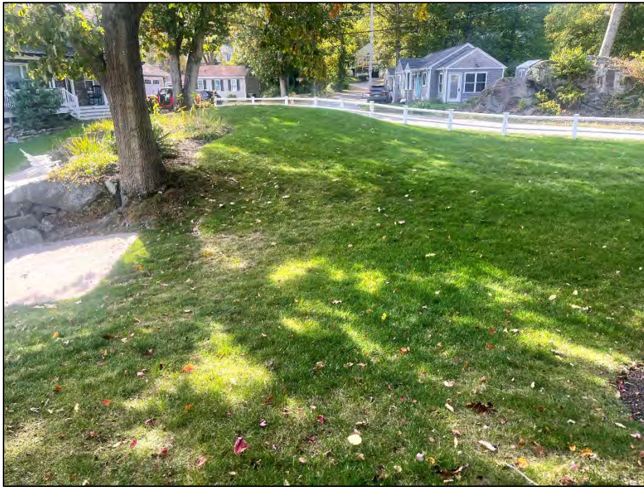
Photo No. 31.: West Dike - Crest as viewed from near STA D0+00 looking left. Note the area of the intentional breach at the left abutment
