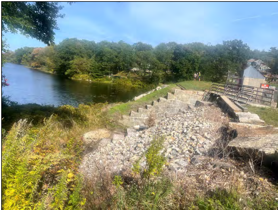
Photo No. 10.: Downstream slope as viewed from the left abutment looking right.
