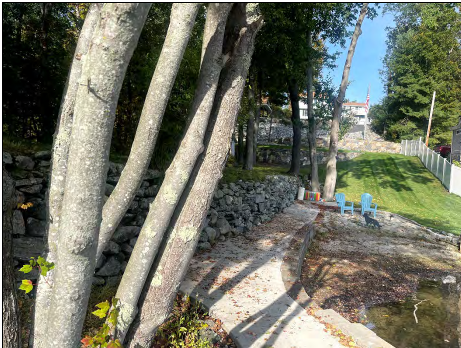
Photo No. 30.: West Dike - Upstream side as viewed from near STA 1+75 looking right.
