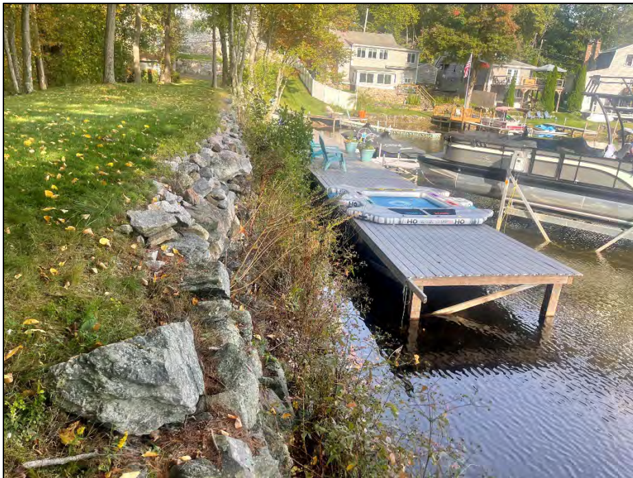
Photo No. 28.: West Dike - Upstream side as viewed from near STA 0+90 looking right.
