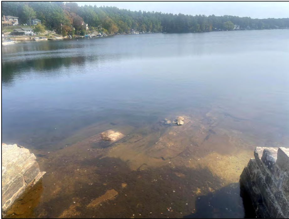
Photo No. 25.: Impoundment as viewed from the primary spillway approach. Note bedrock along the approach below water.
