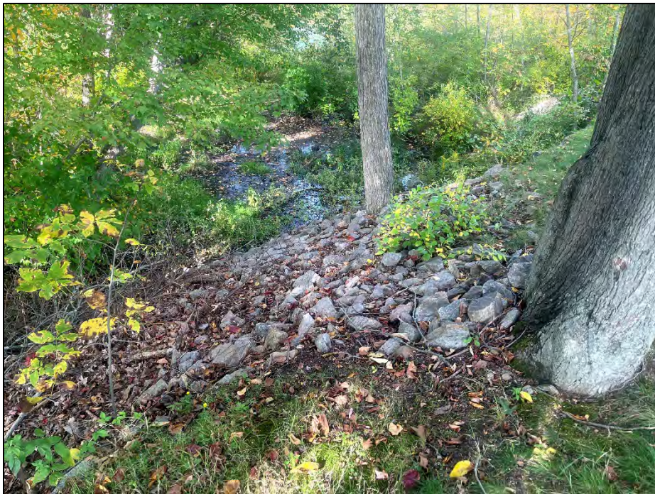
Photo No. 36.: West Dike - Downstream side as viewed from near STA D0+90 looking right. Note the trap rock buttress.
