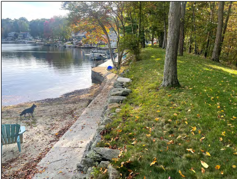
Photo No. 34.: West Dike - Crest as viewed from the right abutment looking left.
