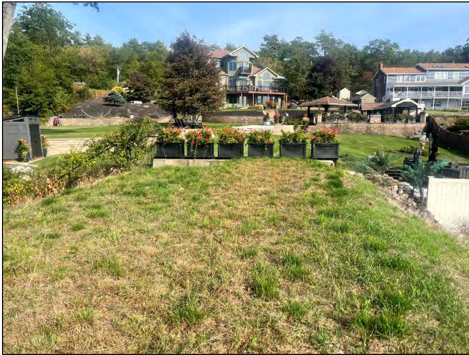
Photo No. 9.: Overview of the crest looking towards the right abutment as viewed from near STA 4+10 looking right.
