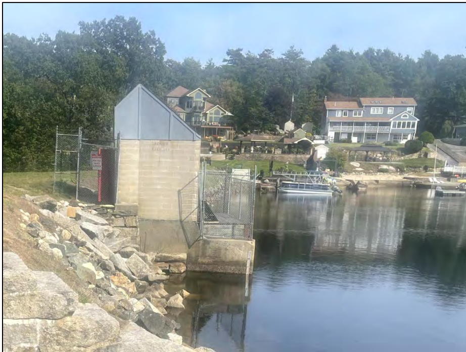
Photo No. 20.: Low level outlet structure as viewed from the primary spillway looking right.
