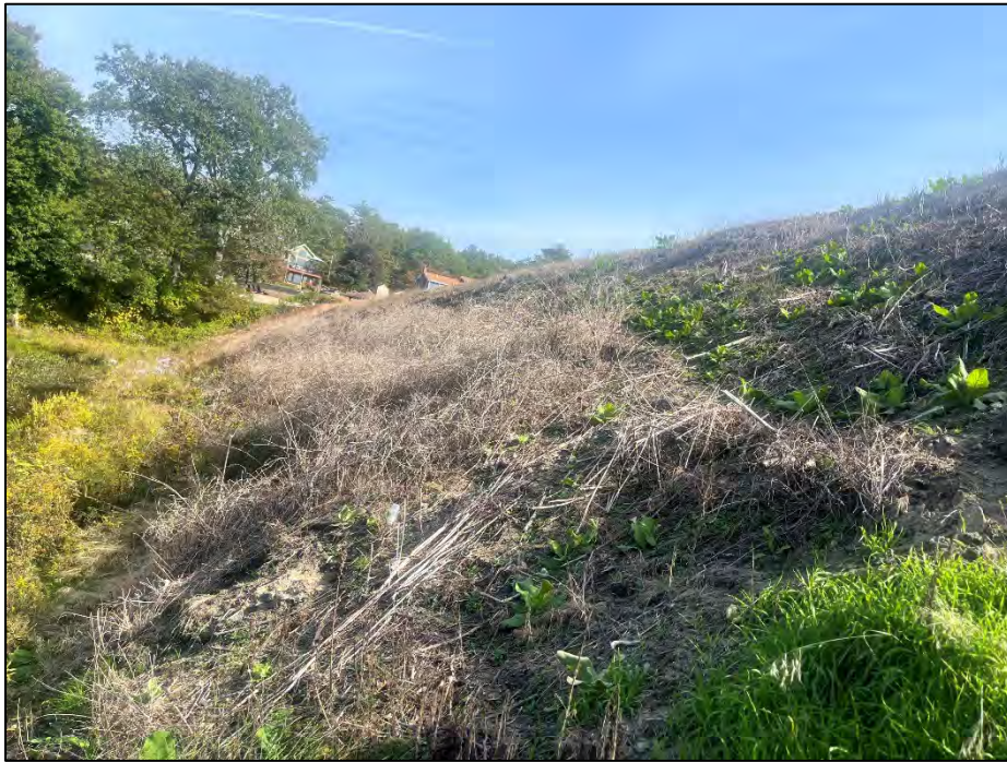
Photo No. 13.: Downstream slope as viewed from right of the low level outlet looking right. Note the steep slope, and the damp and soft toe as identified by the greener vegetation.
