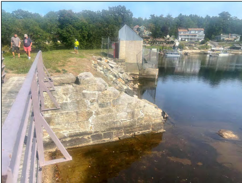
Photo No. 18.: Primary spillway upstream right wall.
