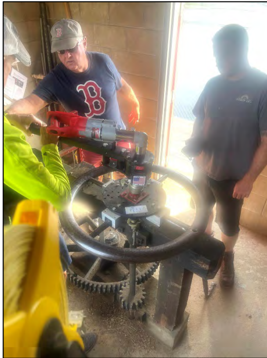
Photo No. 21.: Caretakers demonstrating the operability of the low level outlet gate. Photo looking upstream and slightly right.
