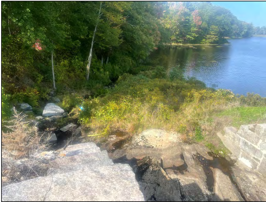
Photo No. 19.: Primary spillway discharge channel.
