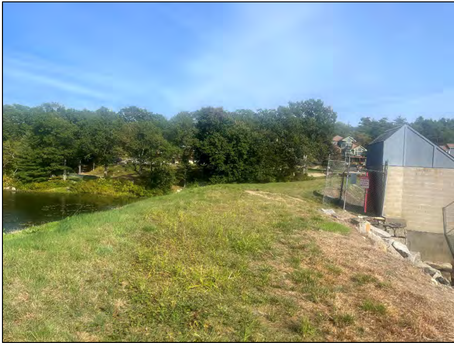
Photo No. 7.: Crest as viewed from right of the primary spillway looking right.
