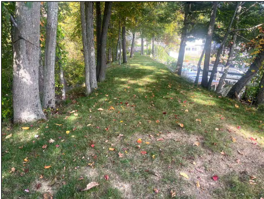
Photo No. 32.: West Dike - Crest as viewed from near STA D0+00 looking right.
